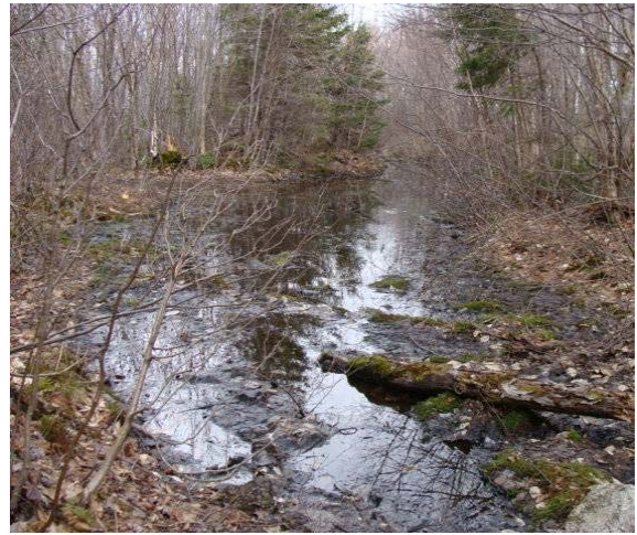
Ponded depressions in a woods road.
