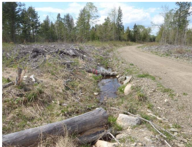
Wet road ditch.
